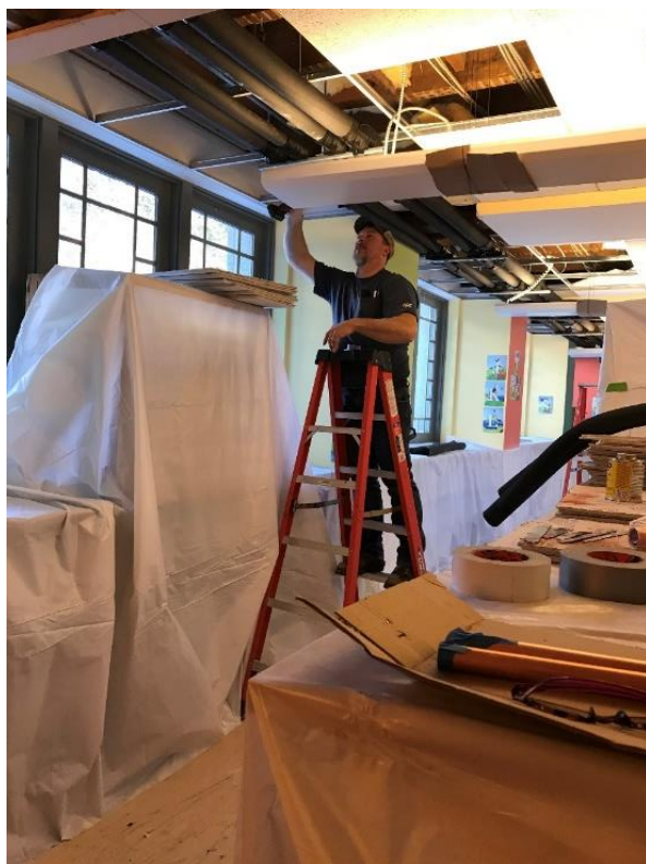
ARC Mechanical's Ray LeClair works in the library's lower-floor ceiling to install brand new refrigeration pipes.
